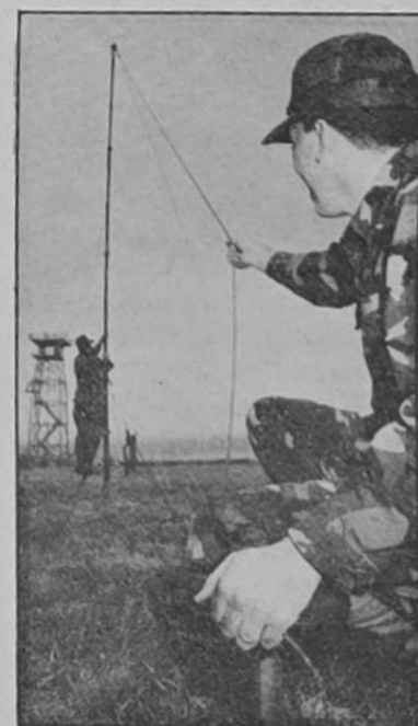
SSgt. Jeffery Smeby and A1C Jimmy Odem (right) erect the 12-meter telescopic antenna mast, a component of the QRCT at 3WW's Det. 16, 9WS. (U.S. Air Force photo)
