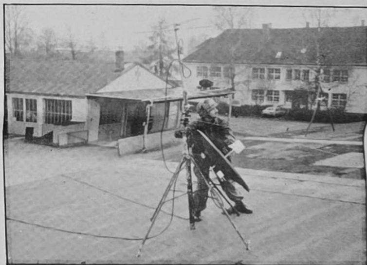
SrA. Randolph Rodriguez adjusts the WRAASE satellite dish on top of the roof of an empty German warehouse.
