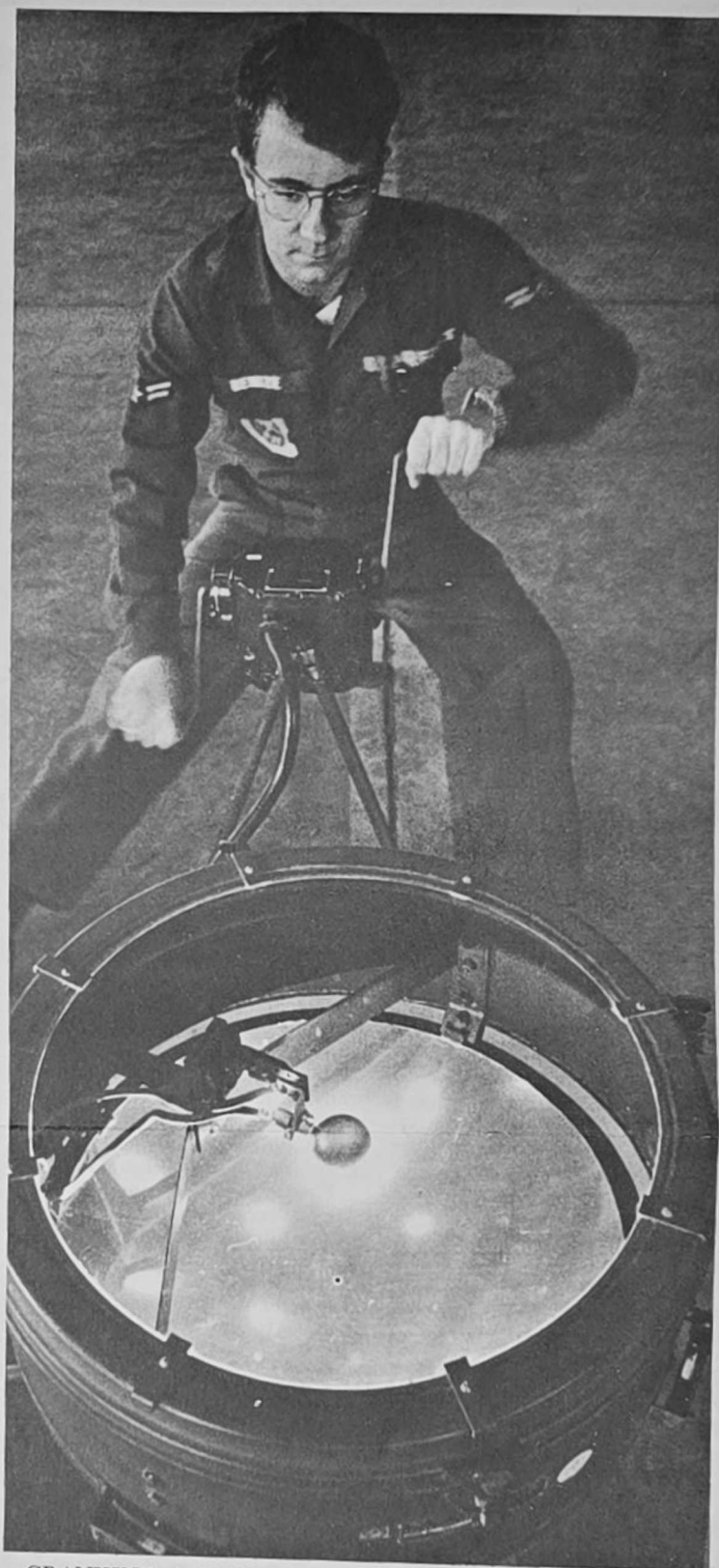
CRANKING A GENERATOR that puts the ceilometer to work is A1C Dennis W. Henize. The TMQ-2 ceilometer, which looks like a huge spotlight, is used to determine cloud heights.
