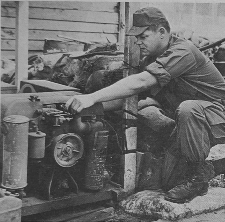
AUXILIARY POWER is a must in the Republic of Vietnam and SSgt. Robert E. Van Buren Operating Location 3, 5th Weather Squadron, Phu Loi Airfield, South Vietnam, is insuring that his unit's generator will not fail by making a spot check of the generator's moving parts.
