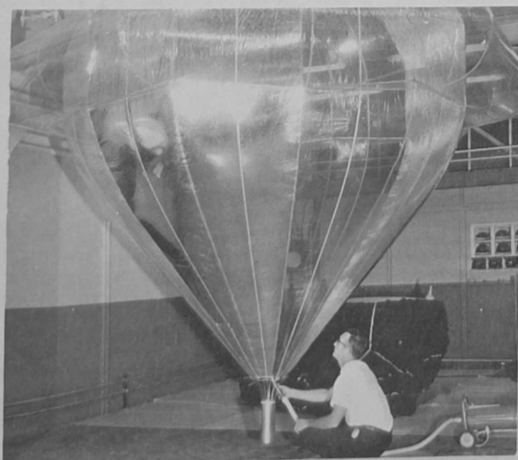
An experimental ballute is being tested at AFRCL. The ballute might eventually replace the weather parachute so that more reliable soundings might be obtained from weather rocketsondes.
