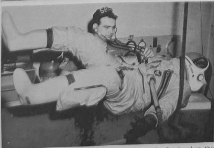
SINCE A SUIT MALFUNCTION could easily be fatal, when the suit is out of commission the mission is scrubbed. MSgt. George T. Davidson, a personal equipment specialist, listens carefully for air leaking from an inflated suit. He checks the high altitude gear prior to each flight.
