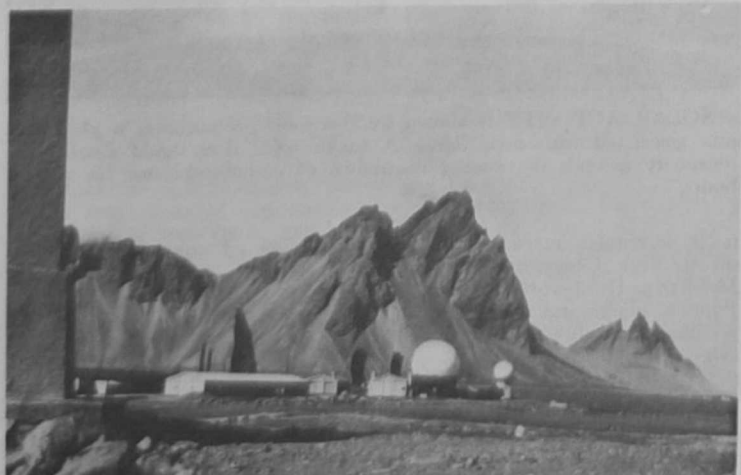
RADAR ANTENNAS probe skies over polar regions to detect manned bomber or missile forces which may choose the polar route. This site is one of a number of radar sites located along the Arctic region. The chain of radar sites, called DEW Line, is located along the Arctic Circle stretching from the Aleutian Islands to Greenland. The entire line covers a distance of nearly 5,000 miles and is divided into eight operational sectors.
