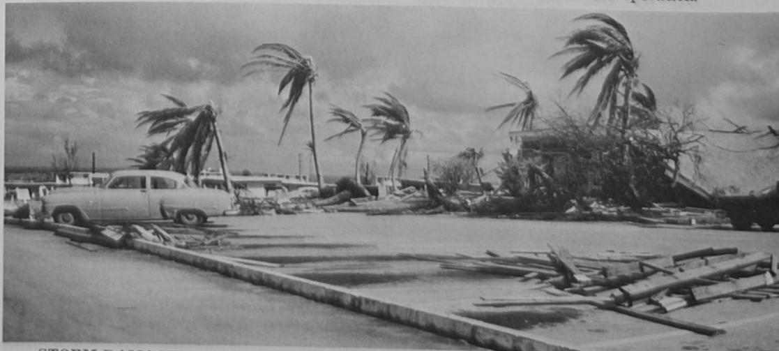
STORM-DAMAGED buildings presented a scene of devastation following Typhoon Karen which struck Guam in 1962. WESTAF aircraft evacuated more than 750 servicemen, women and children to the mainland as part of the MATS relief effort.
