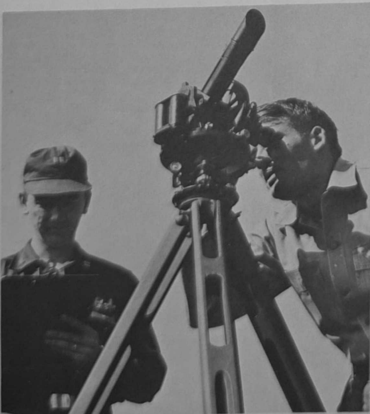
PILOT BALLOON is followed by A2c David H. Jones through a theodolite to determine wind velocities at Mikra, Greece, as Capt. John F. Morrisette (left), records the findings.
