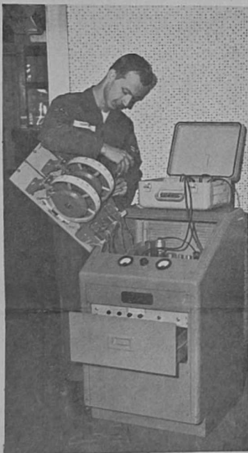
PREVENTATIVE MAINTENANCE is performed on the TMQ/11 temperature-humidity measuring set by Detachment 7's maintenance specialist A2c Terry N. Thompson.
