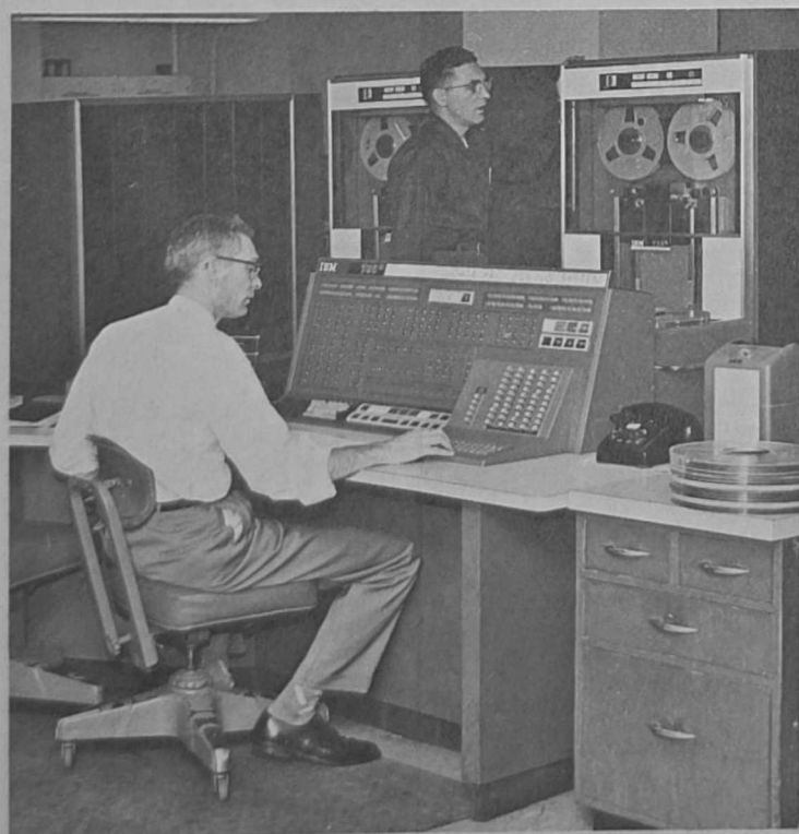
AWS GLOBAL RECORDS are processed on the 705-III Electronic Data Processing System by Frank Taylor (at the console), and Harrell C. Hoglen (at the tape drive), as they start a run, transferring global data from tapes to punch cards.
