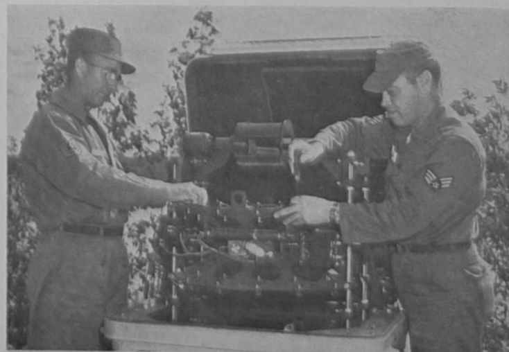
ADJUSTING THE REFLECTOR on the RBC at Galena AFS, Alaska, are TSgt Purfy J. Melebeck, left, and A/1c Martin A. Powers, of the 11th Weather squadron's Field Maintenance shop.
