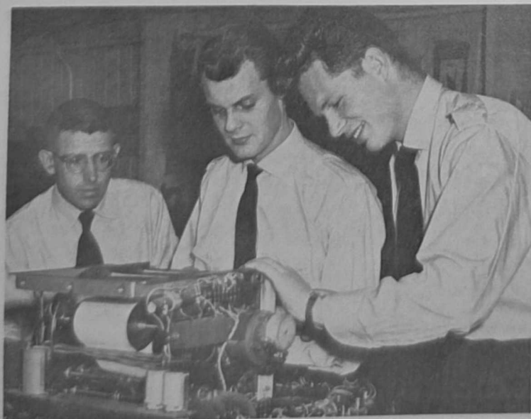
TWO ROYAL DANISH Air Force sergeants work on an AN/GMD-1A under the supervision of TSgt Robert Young, in the 18th Weather Squadron field maintenance shop as part of their five-week course there. The GMD-1A is used globally by AWS to track an airborne radiosonde transmitter to make use of its weather data. The airmen, studying in the Wiesbaden, Germany, unit under the Military Assistance program, are MSgts Paul E. B. Joergensen and Gunnar C. Knudsen.
